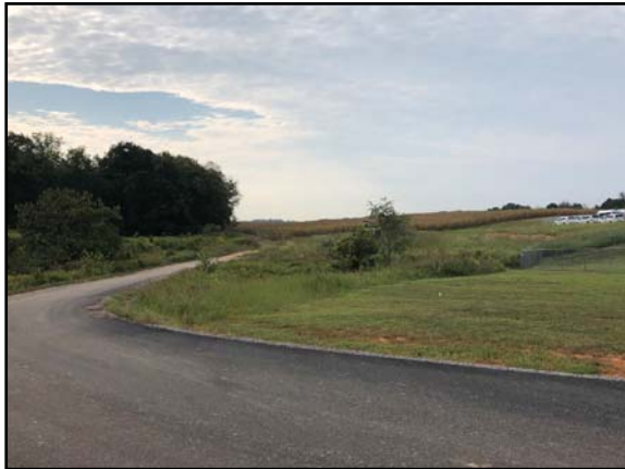
Photo 1. View of the north side of the site with the existing asphalt paved road and surface depression (facing southeast)
